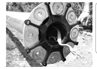
IMPORTANT: Install the Skylevel "spider" on the tower top prior to connecting the power wires to Skystream yaw. The wires must pass through center of "spider" as shown in accompanying photograph.
