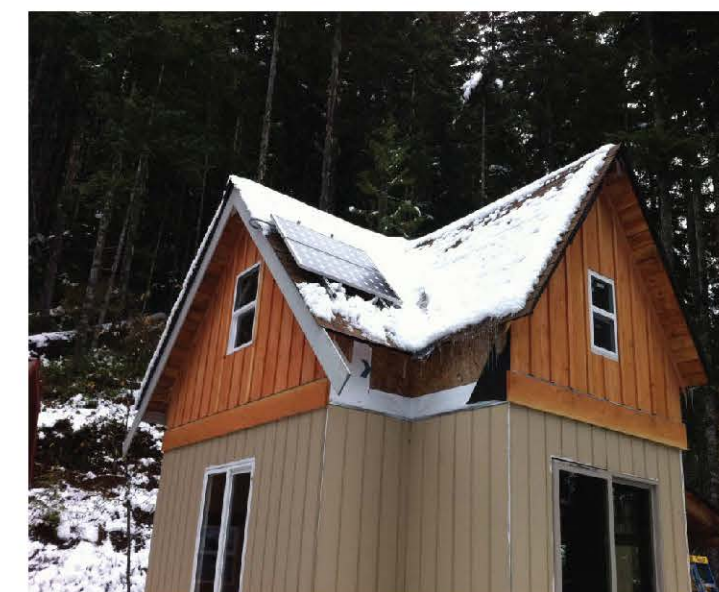
0.5kW Off-Grid PV
